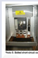
Photo 5: Bolted short-circuit connection for MCCB + N
